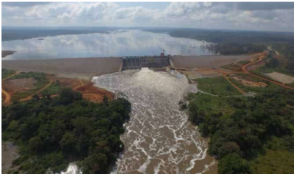
喀麦隆隆潘卡尔水电站建设项目 Lom Pangar Hydro-Power Station in Cameroon
