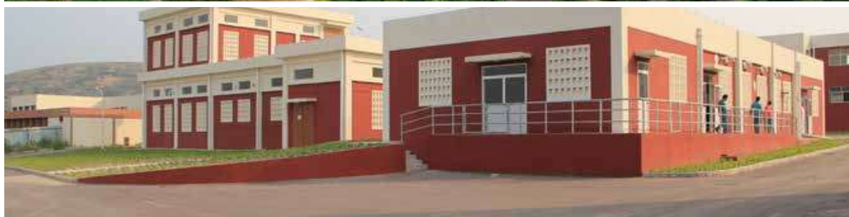
刚果（布）吉利水厂项目 Djiri Water Plant Project in the Republic of Congo
