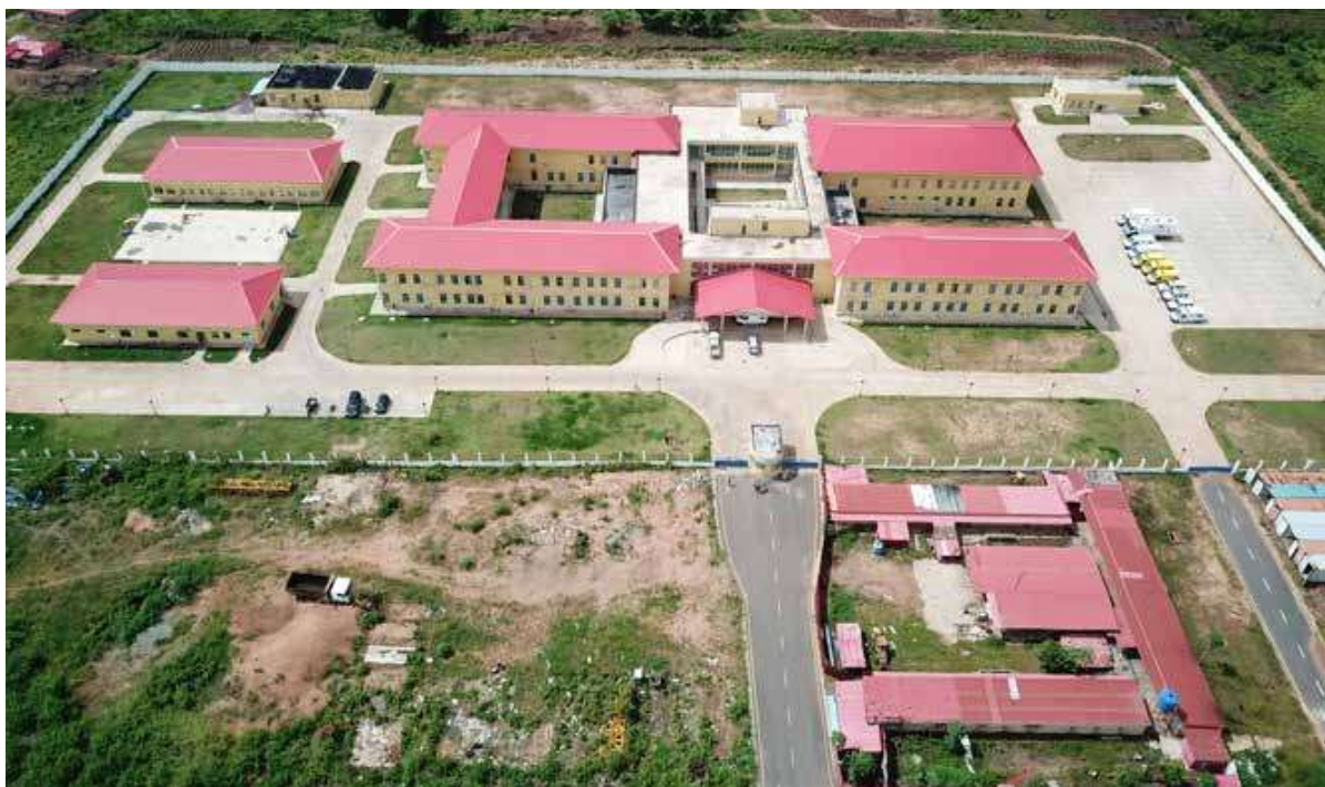
安哥拉北隆达敦多市妇幼医院建设项目 Construction Project of Maternal and Child Hospital in Dundo, North Lunda, Angola
