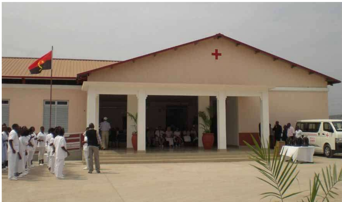
安哥拉学校、医院建设项目一期 Schools and Hospitals Construction Project in Angola, Phase I
