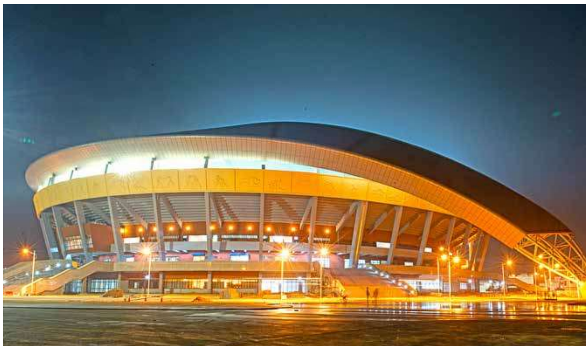
非洲第一座现代化摔跤场—塞内加尔竞技摔跤场 First Modern wrestling ground-Project of Sports Wrestling Field in Senegal
