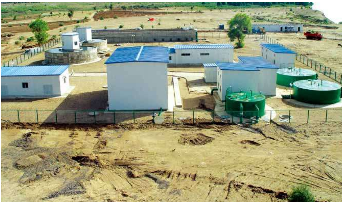
苏丹马兹穆供水项目 Mazmoom Water Supply Project in Sudan
