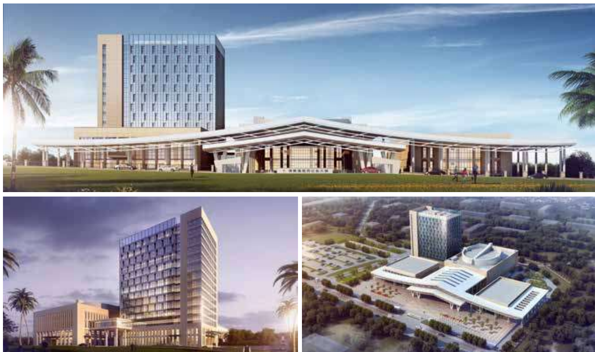
援喀麦隆国民议会大楼项目 Aid Cameroon National Council Building Project
