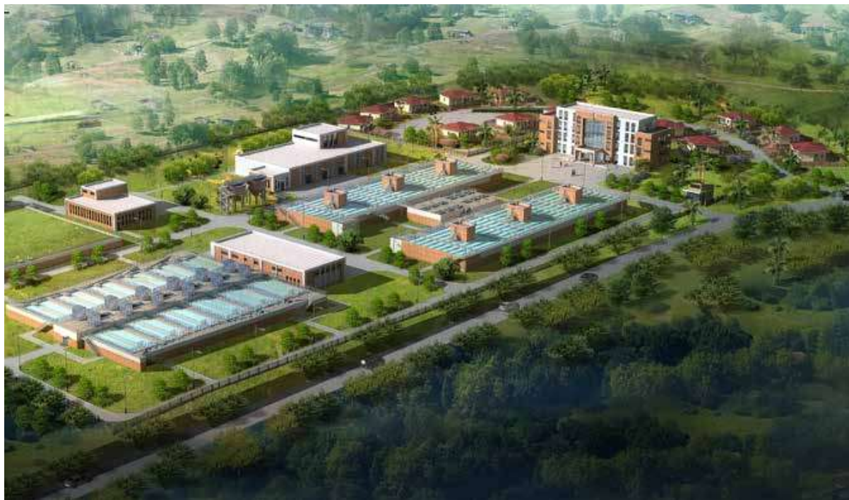
非洲中西部最大污水处理厂——喀麦隆雅温得市萨纳加饮用水处理厂 Africa's largest sewage treatment plant in the Midwest-Sanaga DWTP Project in Yaounde of Cameroon
