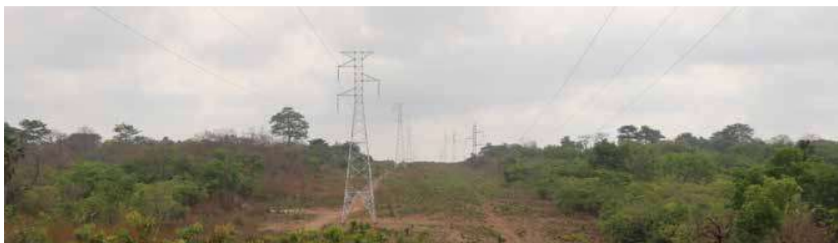
集团本部开拓的第一个非洲输变电项目——科特迪瓦电网改造项目 SINOMACH Headquarters' First Power Transmission Project in Africa - Electric Network Development and Rehabilitation Project of Côte d'Ivoire
