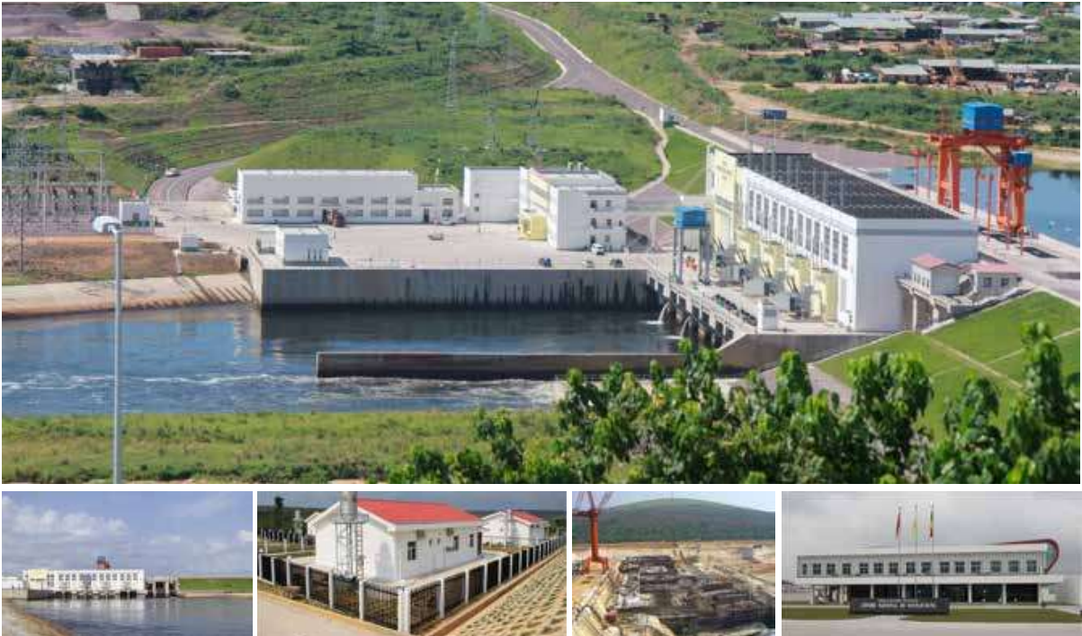
刚果（布）英布鲁 120MW 水电站及配套输变电项目 120 MW IMBOULOU Hydro Power Plant And Associated Transmission Lines Project in the Republic of Congo
