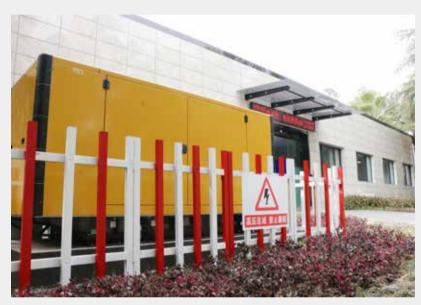
飞轮储能不间断电源系统(飞轮 +UPS+ATS)和柴油发电机组 Flywheel Energy Storage Uninterruptible Power Supply System (Flywheel+UPS+ATS) and diesel power generator set
