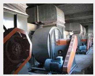
排风及过滤系统 Air Exhaust and filtration system
