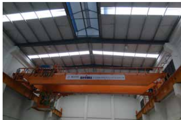
粤丰环保集团横沥项目—汽机房电动双梁吊钩桥式起重机 Waste-to-Energy Project in Hengli Dongguan, China—Turbine Room Crane
