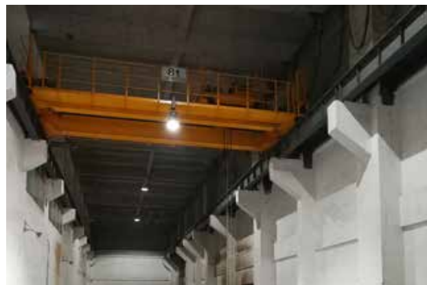
宜宾市生活垃圾焚烧发电项目—灰渣抓斗起重机 Waste-to-Energy Project in Yibin, China—Slag crane
