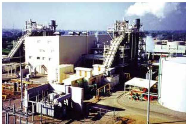
巴基斯坦 KAIRWALA 燃气蒸汽联合循环电站装机容量 2x50MW 燃气轮机 + 44MW 蒸汽轮机 + 2x110t 余热锅炉 KAIRWALA Combined Cycle Power Plant, Pakistan Installed capacity 2x50MW gas turbine + 44MW steam turbine + 2x110t waste heat boiler
