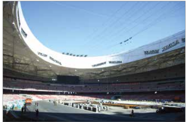
国家体育场（鸟巢）顶部威亚承载钢索系统 Wire bearing steel cable system on the top of National Stadium (Bird's Nest)
