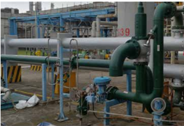
茂名石化公司发夹式高压换热器 Hairpin-type high pressure heat exchanger of Sinopec Maoming Petrochemical Company
